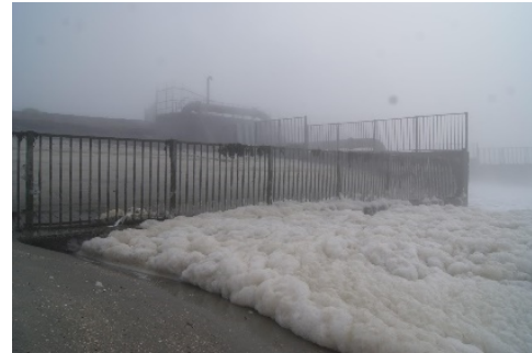
Fig. 4: Area behind the power plant where the cooling water is led back into the sea (11.01.2022).
